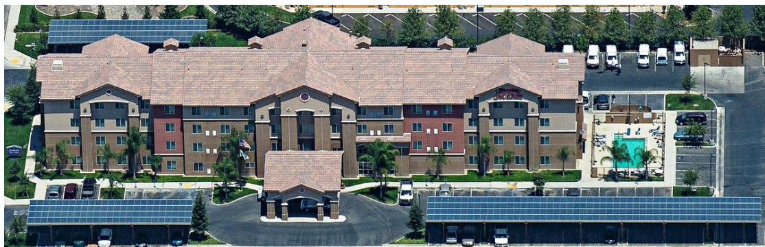
Figure 7. Hotel Hampton Inn in California with photovoltaic installation
